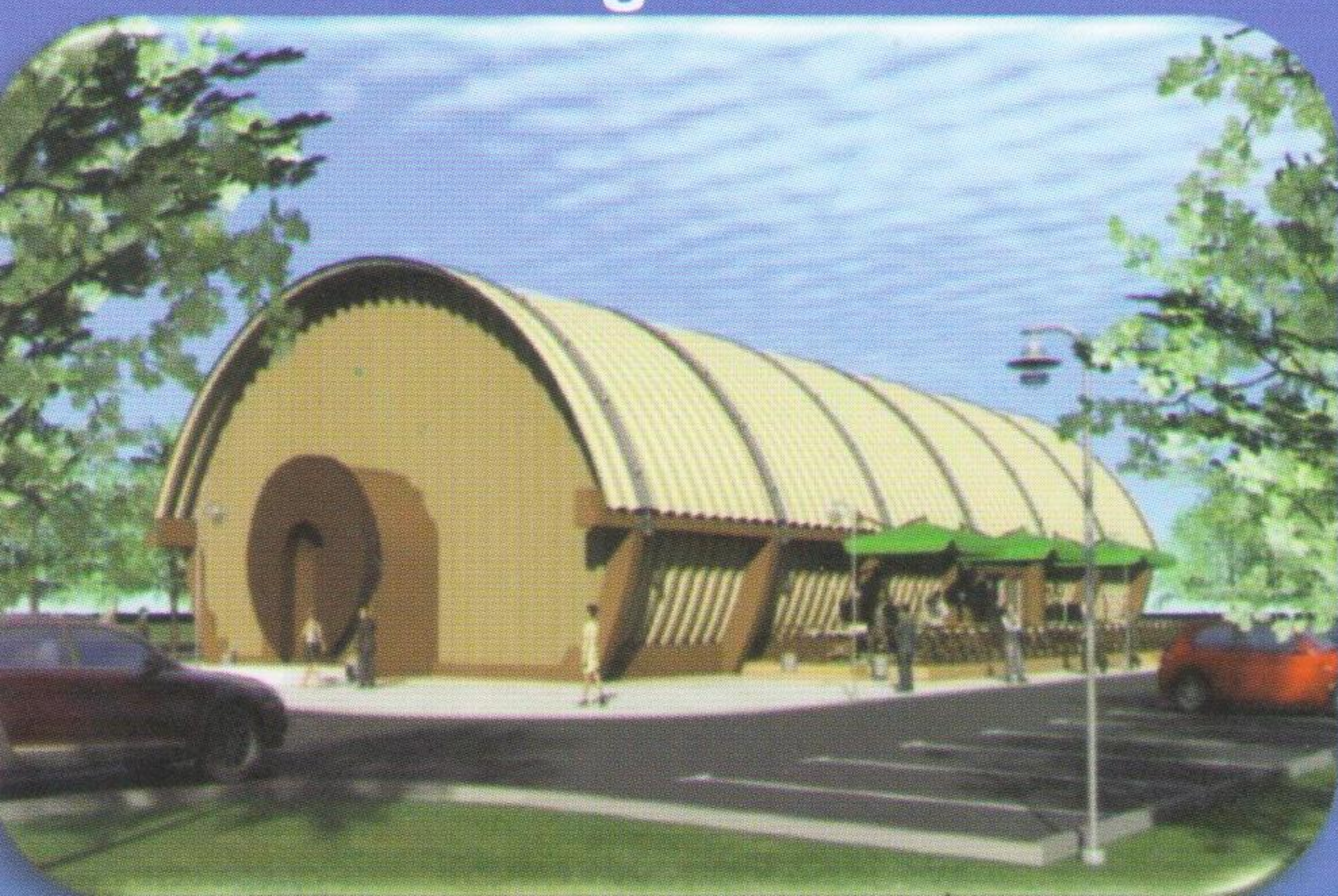
Frameless Arch-Type Building Variant
